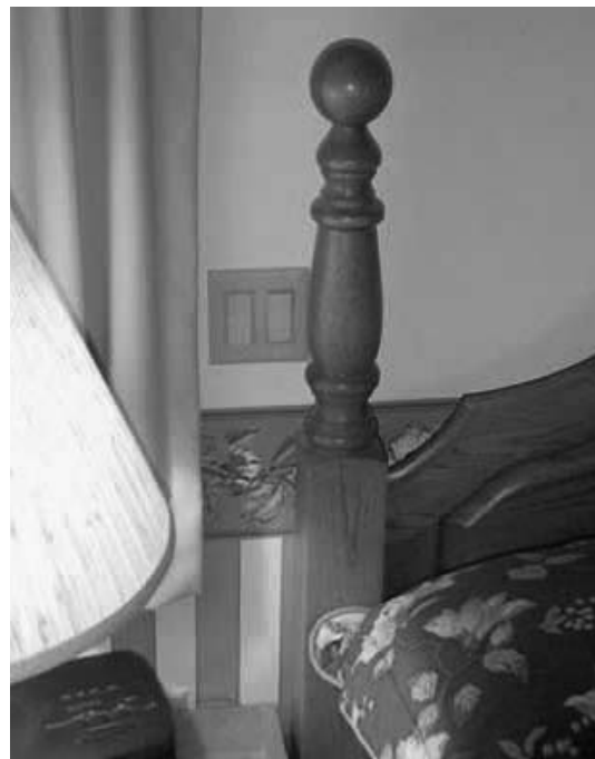
Rocker light switches reachable from the bedside, located 36" to 40" above the floor.
